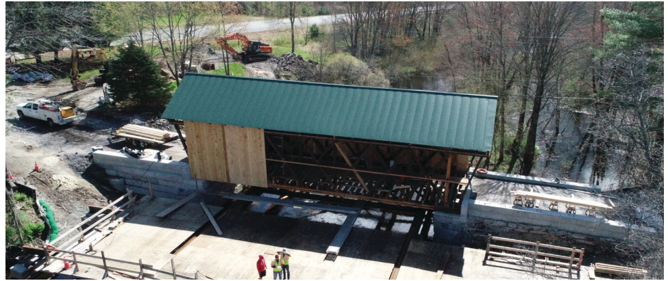
Aerial view of siding installation, May 6, 2021.
