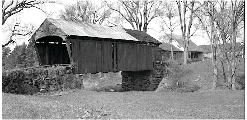
Looking from the south toward what is now Route 103, a railroad crossing can be seen on the right. Weather damage to the siding and roof are obvious, likely caused by the great hurricane of 1938. This is one of oldest photos of the Bridge taken in 1939.
