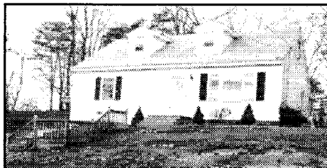
#1542 CONCORD: Three bedroom Cape in great neighborhood, new furnace, tile floor in kitchen, maple cabinets, wood floors, great fenced back yard, family room in basement, motivated seller. $255,000
